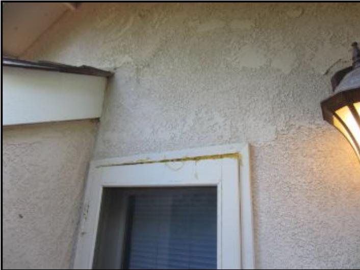
Bathroom exterior door with expanded foam seal
